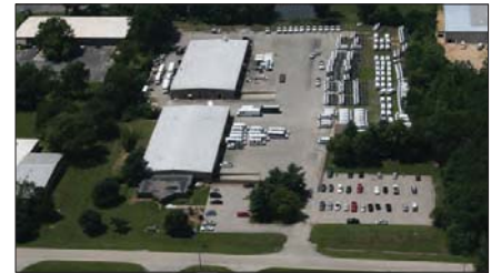
2503 Ada Dr., Elkhart 44,295 SF in 2 buildings. 8.69 acres. Fenced. Many docks and o/h doors, 16' eaves. Sale Price: $1,450,000 Bill Kuhns, SIOR
