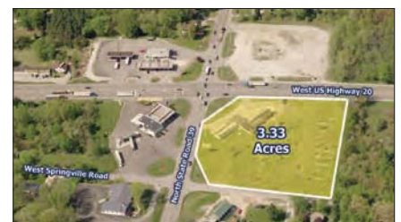
1838 US Hwy. 20, LaPorte 3.33 acres. Private well/septic system. Highly visible with good traffic count. Zoned B-2. Offered at: $595,000 Pete Letherman, SIOR, CCIM
