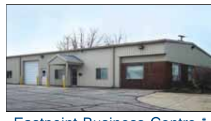
Eastpoint Business Centre * 2701 Industrial Pkwy., Elkhart Newly renovated multi-tenant building Flex space: 2,056 SF & 2,154 SF Lease: $4.00-$5.50 PSF Carl Tiedemann, SIOR
