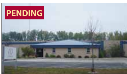
2135 Industrial Pkwy., Elkhart 78,132 SF, 4.48 acres. 18' ceilings. Features eight docks & three overhead doors. Zoned M-1. Lease: $2.50 PSF Pete Letherman, SIOR, CCIM
