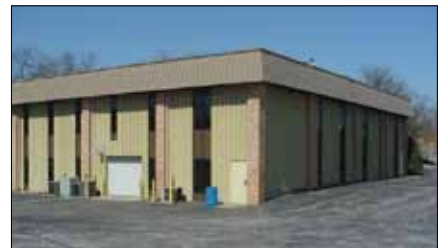
1010 N. Main St., Elkhart Two buildings. 51,246 SF on 2.99 acres. Fenced property. Sale Price: $495,000 Brent Miller, SIOR
