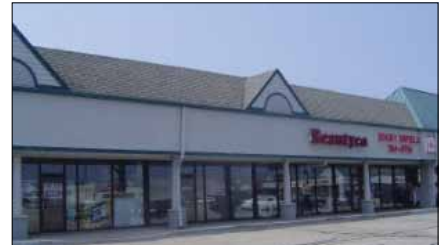
Northview Dr., Elkhart North Pointe Retail Center. Anchored by Kmart. Close to hotels & restaurants. Call for pricing. John Letherman, CCIM
