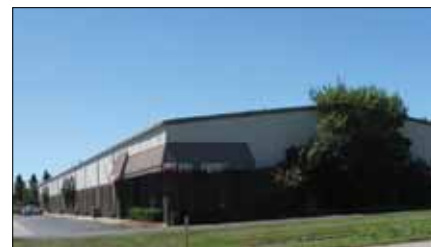
53042 Faith Ave., Elkhart 6,000 SF unit available. Has dock & overhead door. 16' ceilings, clear span. Lease: $3.00 PSF Bill Kuhns, SIOR
