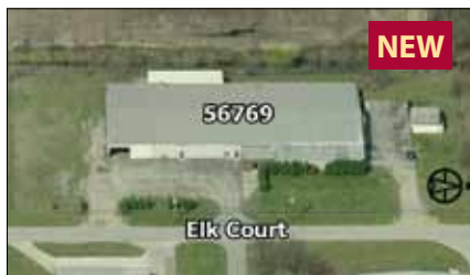
56769 Elk Court, Elkhart 27,949 SF total includes 20,000 SF steel building & 520 SF office. 3 o/h doors, 3-Phase. Sale price: $450,000 Scott Griffith/Bill Kuhns, SIOR
