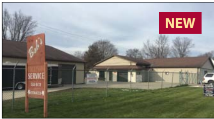
805 & 815 S. Ninth St., Goshen 12,132 SF 3-building complex on 0.75 acres with 8 o/h doors and 8' to 14' ceilings. Offered at: $265,000 Scott Griffith
