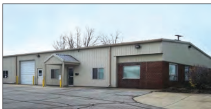
Eastpoint Business Centre * 2701 Industrial Pkwy., Elkhart Newly renovated multi-tenant building. Flex space: 2,056 SF & 2,154 SF Lease: $4.00-$5.50 PSF Carl Tiedemann, SIOR
