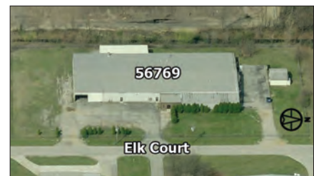
56769 Elk Court, Elkhart 27,949 SF total includes 20,000 SF steel building & 520 SF office. 3 o/h doors, 3-Phase. Sale price: $450,000 Scott Griffith/Bill Kuhns, SIOR
