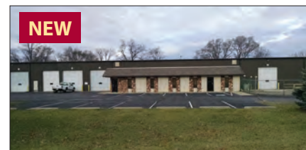
NEW 29221 CR 20, Elkhart 22,312 SF on 2.69 acres. Eight 14' o/h doors, 1 dock, one 2-ton bridge crane, several 1-ton jib cranes, 3-phase power. Lease: $3.12 PSF Bill Kuhns, SIOR
