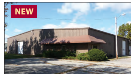
NEW 3608 Cooper Drive, Elkhart 21,500 SF with 6 o/h doors, 1 dock, 16' ceilings, heavy power, roof coated 2015. Lease: $2.76 PSF Brent Miller, SIOR
