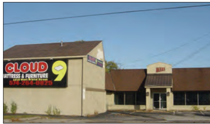
1220 W. Bristol St., Elkhart 21,509 SF building on 1.44 acres. 158' frontage on busy Bristol Street. Sale Price: $150,000 Pete Letherman, SIOR, CCIM
