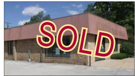
952 E. Jackson Blvd., Elkhart 11,989 SF. 4,789 SF warehouse space, full basement with lift & 7,200 SF showroom. SOLD 3Q 2015 John Letherman, CCIM
