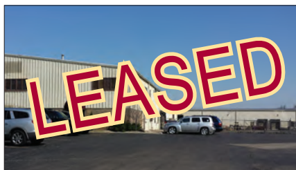
3604 Cooper Drive, Elkhart 2 buildings totaling 34,000 SF. 4 o/h doors, 4 docks. LEASED 4Q 2015 Ross Miller, SIOR Brent Miller, SIOR
