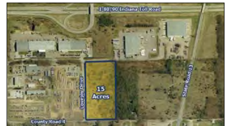
CR 4 & Lovejoy Dr., Middlebury 15 acres. Adjacent to former IBS buildings. Zoned M-2. Offered at: $297,400
