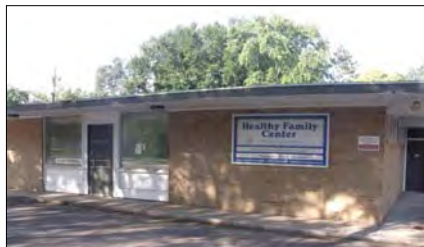
603 Oakland Ave., Elkhart 2,496 SF. 6 offices/exam rooms, reception area, 2 waiting areas. Lease: $5.00 PSF. Sale Price: $59,900 Richard Hobson
