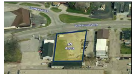
1609 W. Bristol St., Elkhart 0.69 acres. Good visibility in high traffic location. Zoned B-3.
