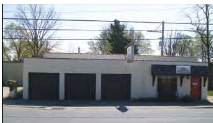
102 Charles St., Bristol 4,000 SF with office, 4 overheads, 14' ceilings, small paint booth. Lease: $2.85 PSF. Sale Price: $119,900 Richard Hobson
