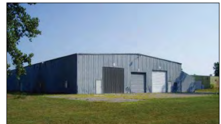
19875 M-205, Edwardsburg 19,690 SF on 6.3 acres. 16'-18' ceilings, 3 overhead doors, fenced yard, security system. Sale Price: $510,000 Ross Miller, SIOR
