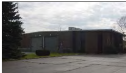
109 14th St., Middlebury Former Pilgrim International 54,700 SF with 22' ceilings, 35 overhead doors. Lease: $3.00 PSF Pete Letherman, CCIM
