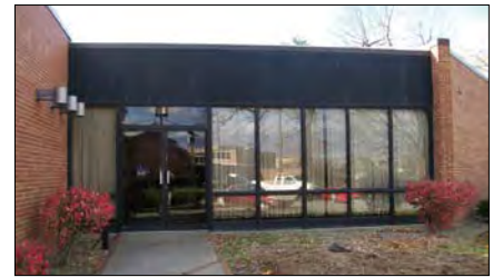
327 W. Marion St., Elkhart Former Social Security Office 7,052 SF with new carpet, paint and windows. Lease: $5.00 PSF Richard Hobson
