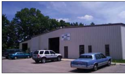
52782 Lillian St., Elkhart 10,000 SF on 1 acre. 3 overhead doors, 3-Phase power, 24'x 40' column spacing. Lease: $3.36 PSF Bill Kuhns, SIOR
