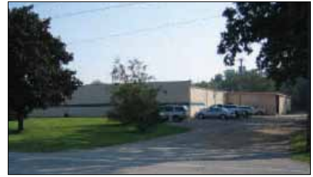
806 S. Division St., Bristol 20,000 SF. 16'-20' ceilings, 2 docks, 6 overhead doors, high intensity lighting. 1,000 SF office. Sale Price: $299,000 Brent Miller, SIOR
