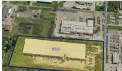
West Hively Ave., Elkhart 205,800 SF building. Fully leased. 13.7 acres. 22' ceilings. 5 docks & 5 overhead doors. Call for pricing. Pete Letherman, SIOR, CCIM
