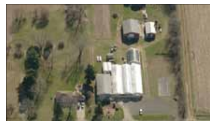
51538 CR 19, Bristol 35 acres of land with six commercial buildings and 2,614 SF house. Lots of possibilities! Sale Price: $395,000 John Letherman, CCIM
