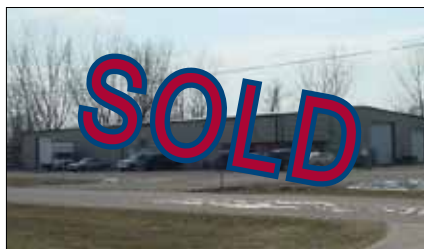
2933 Paul Dr., Elkhart Former Damon Plant 8 is 12,000 SF. 25'x 40' bays. Airlines, fenced. SOLD 1Q 2013 Brent Miller, SIOR
