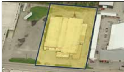
1700 W. Lusher Ave., Elkhart 40,000 ± SF. Very good condition, new roof in 2009. 5 overhead doors & 1 dock. Sale Price: $650,000 Ross Miller, SIOR
