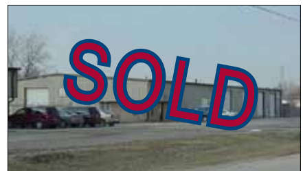
2939 Paul Dr., Elkhart Former Damon Plant 12 is 14,000 SF. 25'x 40' bays. SOLD 1Q 2013 Brent Miller, SIOR
