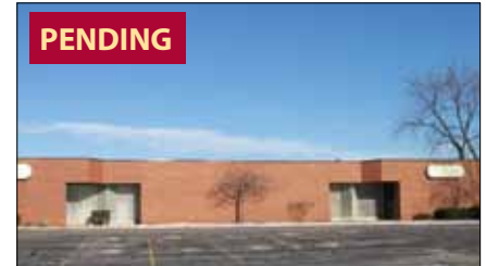
501 Wall St., Valparaiso 8,205 SF medical office building. 0.65 acres. Features gym & small therapy pool. Sale Price: $595,000 Richard Hobson
