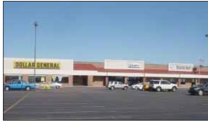
2014 Lincolnway East, Goshen Goshen Commons I. One suite of 8,342 SF remains. Lease: $8.00 PSF Pete Letherman, SIOR, CCIM
