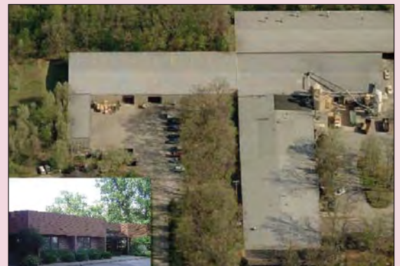
3504 Cooper Dr., Elkhart 102,957 SF with 4,940 SF office space. Situated on 8.73 acres. City water & sewer. Zoned M-2. Lease: $2.70 PSF. Sale Price: $995,000 Pete Letherman, CCIM John Letherman, CCIM
