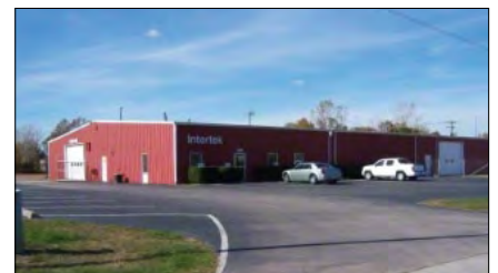
2923 Thorne Dr., Elkhart 712 building has 20,000 SF. ½-Ton crane rail, 2 docks. Lease: $2.76 PSF. Sale Price: $450,000 Bill Kuhns, SIOR
