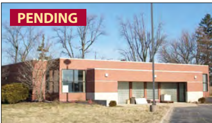
3391 Airport Rd., Portage 5,400 SF medical office building. 0.85 acres. Two front entrances allow for multi-tenancy. Sale Price: $599,000 Richard Hobson
