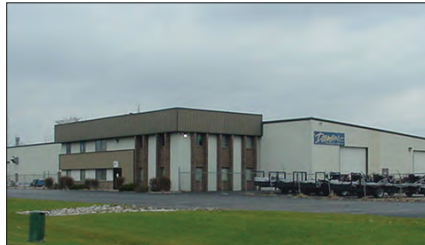
2946 Paul Dr., Elkhart Former Heartland Plant 21. 46,131 SF. 12 overhead doors. 15.25 acres. Sale Price: $895,000 Brent Miller, SIOR
