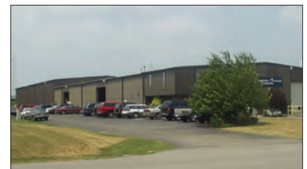
2515 Lombardy Dr., Goshen 30,800 SF. 6.77 acres. Two story office area. Very clean building. 3 docks. 18' eaves. Lease: $2.65 PSF. Ross Miller, SIOR
