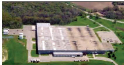
2121 Chicago Rd., Niles Niles Distribution Center. 34,460 & 58,930 SF suites available. 32'4" ceilings. Many docks. Negotiable lease rate. Carl Tiedemann, SIOR Ross Miller, SIOR
