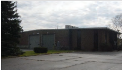
109 14th St., Middlebury Former Pilgrim International 54,700 SF with 22' ceilings, 35 overhead doors. Lease: $3.00 PSF Pete Letherman, SIOR, CCIM
