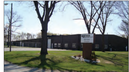
2700 Ada Dr., Elkhart 60,000 SF for lease. 4 docks, 3 overhead doors. 16' eaves. Fenced yard. Zoned M-1. Lease: $2.30 PSF Ross Miller, SIOR
