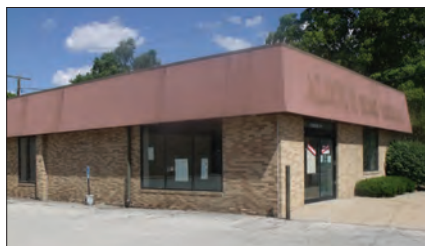
952 E. Jackson Blvd., Elkhart 11,989 SF. 4,789 SF warehouse space, full basement w/lift & 7,200 SF showroom. Lease: $5.00 PSF John Letherman, CCIM
