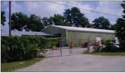
25883 N. Park Ave., Elkhart Former Lee Enterprises. 18,272 SF, 6 overheads. City utilities. Zoned M-1. Sale Price: $195,000 Brent Miller, SIOR
