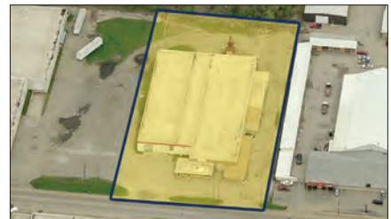
1700 W. Lusher Ave., Elkhart 40,000 ± SF. Very good condition, new roof in 2009. 5 overhead doors & 1 dock. Sale Price: $650,000 Ross Miller, SIOR
