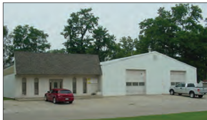
2423 Lowell St., Elkhart Former Hoosier Crane. 8,490 SF. One 5-Ton crane. Lease: $3.00 PSF. Sale Price: $199,500 Brent Miller, SIOR
