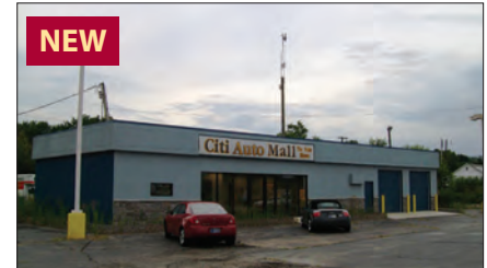
1820 Lincolnway E., South Bend 2,765 SF building on 0.59 acres. Great exposure on busy Lincolnway. 2 OH doors. Sale Price: $368,000 Richard Hobson
