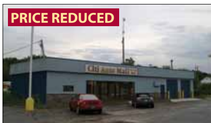
1820 Lincolnway E., South Bend 2,765 SF building on 0.59 acres. Great exposure on busy Lincolnway. 2 OH doors. Sale Price: $330,000 Richard Hobson
