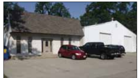
2423 Lowell St., Elkhart Former Hoosier Crane. 8,490 SF. One 5-Ton crane. Lease: $3.00 PSF. Sale Price: $199,500 Brent Miller, SIOR
