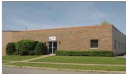
1319 N. Iowa St., South Bend 8,680 SF building on 0.62 acres. Located near South Bend Regional Airport. Sale Price: $265,000 Pete Letherman, SIOR, CCIM
