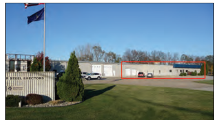
2300 B Johnson St., Elkhart 17,250 SF in shared building with LeMaster Steel on CR 9. Heavy power, 16' ceiling, 2 docks. Lease: $2.80 PSF Carl Tiedemann, SIOR
