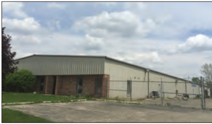
56764 Elk Park Dr., Elkhart 27,000 SF in 2 buildings on 2.5 acres. Heavy power. Mostly clear span. Lease: $2.40 PSF Scott Griffith/Bill Kuhns, SIOR
