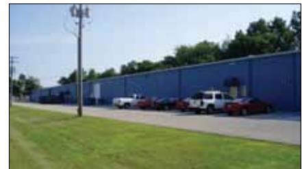
1000 Campus Ct., Elkhart 27,270 SF available. Divisible. 16' ceilings, clear span, 2 overhead doors, 1 dock. Lease: $3.60 PSF Ross Miller, SIOR
