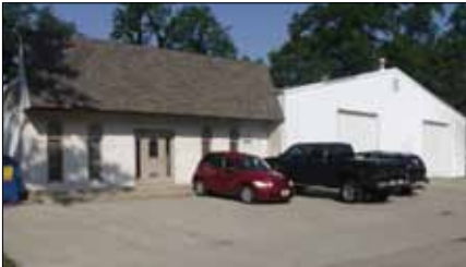
2423 Lowell St., Elkhart Former Hoosier Crane. 8,490 SF. One 5-Ton crane. Lease: $3.00 PSF. Sale Price: $199,500 Brent Miller, SIOR
