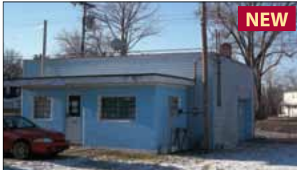
1213 S. Main St., Elkhart 992 SF building. 200 SF office space. Perfect for used car lot or service garage. Sale Price: $80,000 Richard Hobson
